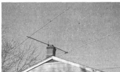
fig. 4. Telescoping section converts a 15-meter dipole to 20 meters. On 20 meters the 15-meter reflector acts as a director.
